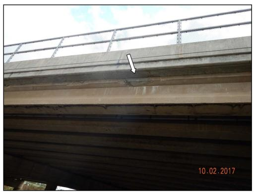
Photo 16: Waukegan Road, beam repair in the top flange, beam 1 in span 3 shown
