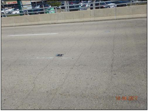
Photo 5: Waukegan Road, typical top of deck map cracking
