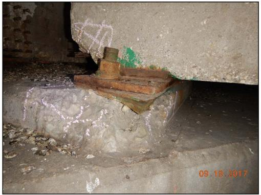
Photo 19: Waukegan Road, unsupported bearing pad and spalled beam seat under beam 8 at pier 2
