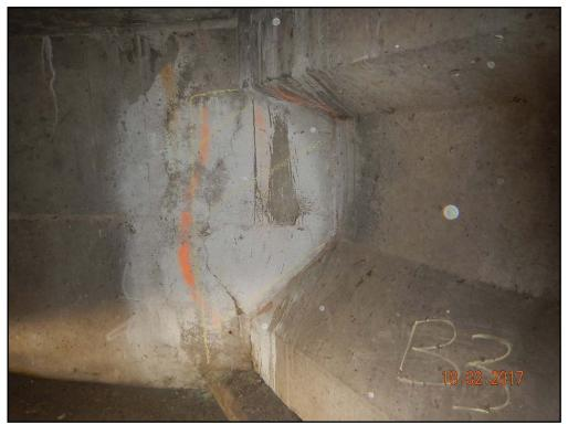
Photo 6: Waukegan Road, typical diaphragm delamination at north abutment (Looking North)
