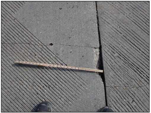
Photo 11: Waukegan Road, spall at south abutment joint
