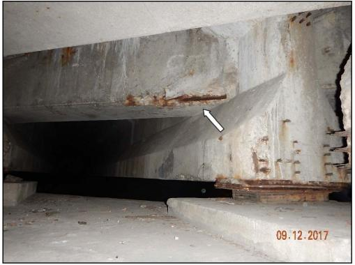
Photo 15: Waukegan Road, typical spalled diaphragm
