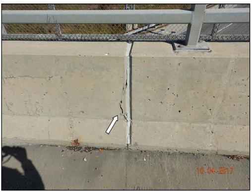
Photo 12: Waukegan Road, typical cracking in the parapet at expansion joints
