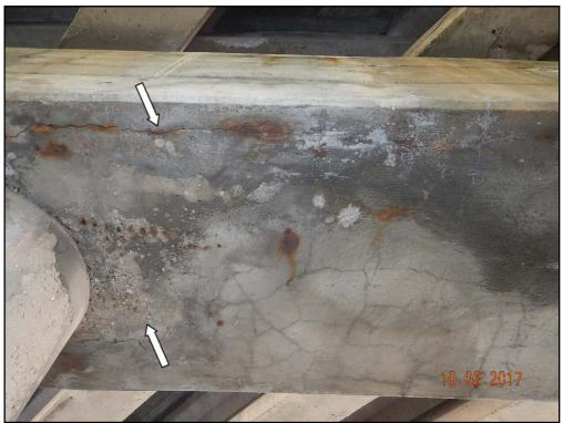
Photo 31: Waukegan Road, scaling and longitudinal cracks with efflorescence on pier 3 cap
