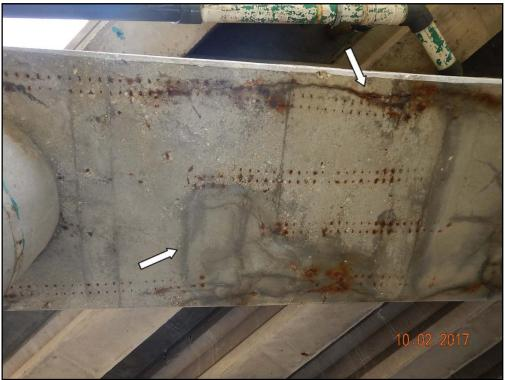
Photo 25: Waukegan Road, typical previous repairs with map cracking and longitudinal cracks with efflorescence, underside of pier 1 cap shown
