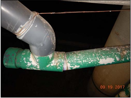
Photo 35: Waukegan Road, loose T-pipe connection in drainage pipe, pier 2
