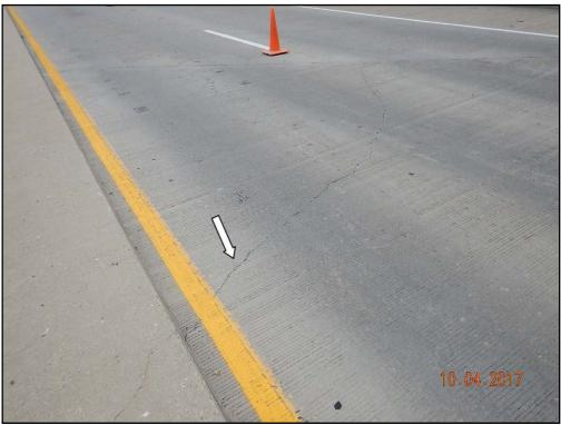
Photo 32: Waukegan Road, intermittent diagonal cracks extending the full length of approach slab, north approach slab shown
