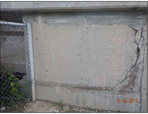
Photo 38: Waukegan Road, typical wingwall spall, northeast wingwall shown
