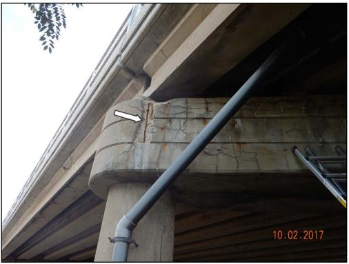
Photo 30: Waukegan Road, spalls with exposed reinforcement on pier 3 cap
