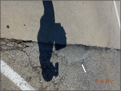
Photo 33: Waukegan Road, asphalt patch in the roadway pavement adjacent to approach slab, north approach slab shown
