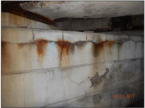
Photo 29: Waukegan Road, horizontal cracks with efflorescence on pier 3 cap
