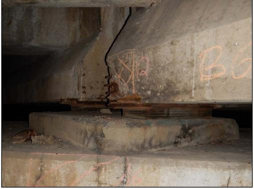
Photo 9: Waukegan Road, typical elastomeric bearing (Looking North)
