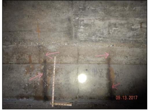
Photo 21: Waukegan Road, intermittent vertical cracks in barrier, pier 1 shown
